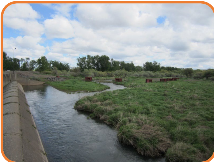
Figure 2-12. Mill Creek Diversion Dam Forebay with Debris Barrier
