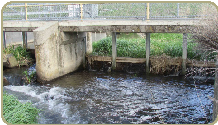
Figure 2-25. Yellowhawk Stoplogs
