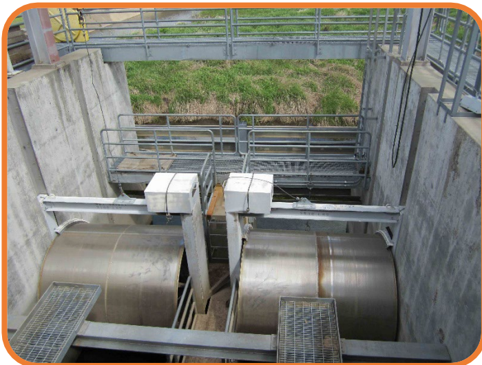
Figure 2-10. Rotating Drum Fish Screens
