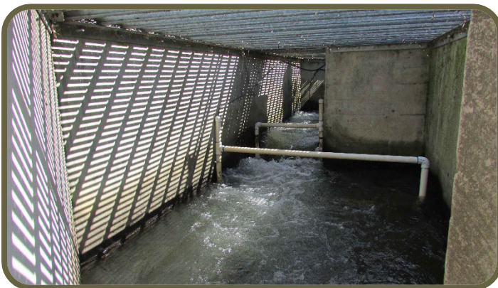
Figure 2-21. Division Dam Fish Ladder
