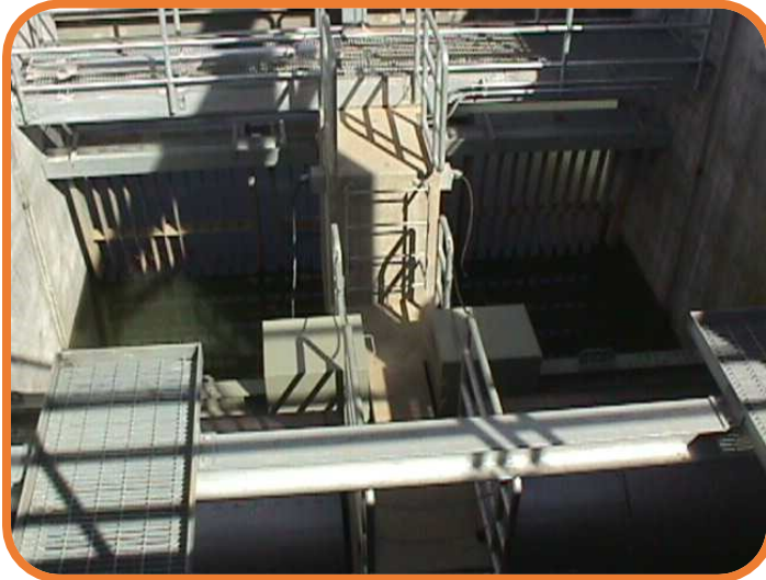
Figure 2-11. Trash Racks in front of Rotating Drum Fish Screens
