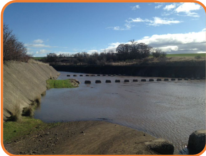
Figure 2-9. Diffuser Blocks in the Intake Canal to Dissipate Energy
